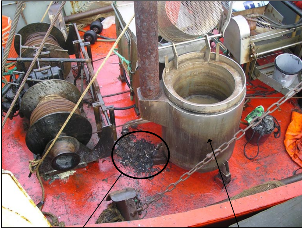
Burnt section of plastic air supply trunking
